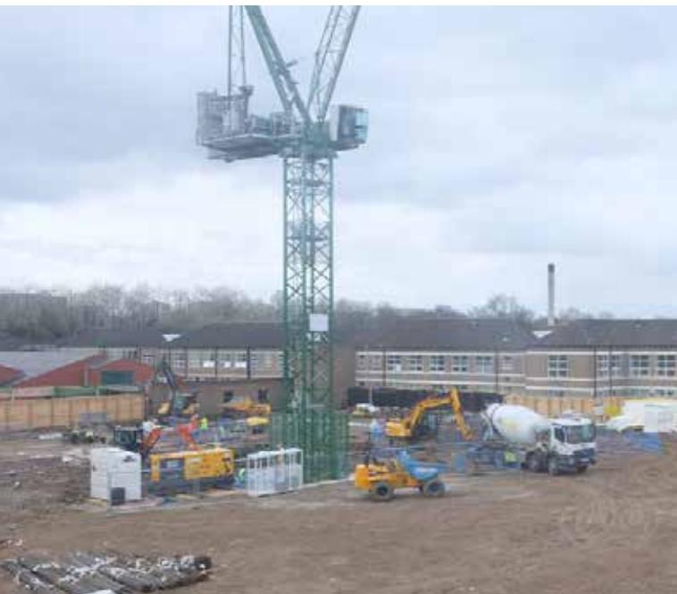
A luffing crane has been erected which will be on site for the construction period. The crane is being used to move steel, concrete and large materials from the loading bay.
